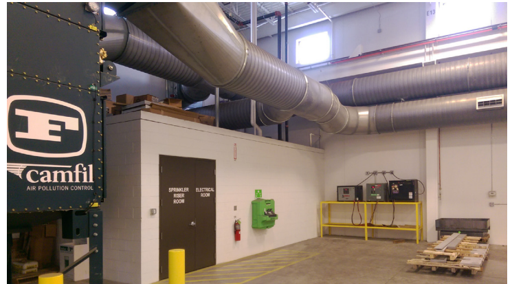
▲ Vented ductwork runs through the entire factory to ensure the circulation of clean air.
