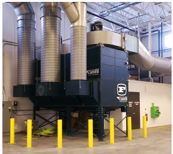
▲ With the Farr Gold Series dust collector, the facility stays clean and clear of dust and fumes.
