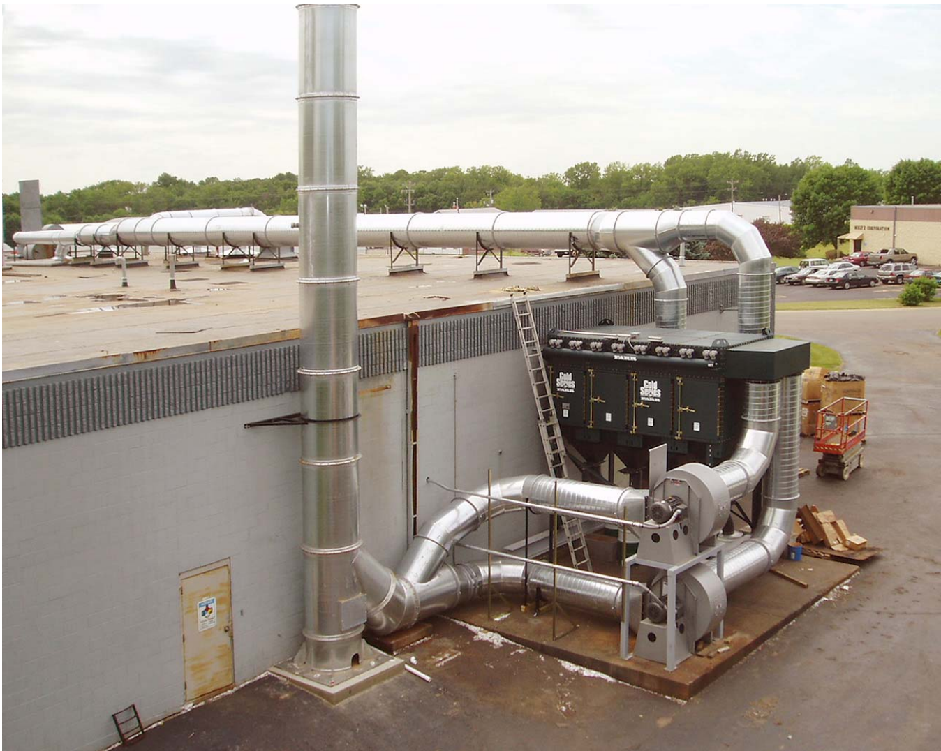
32,000 CFM through the Gold Series provided by twin fans controlled by a variable frequency drive (VFD).
