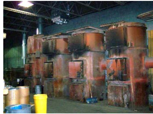
Fumes from incinerators are captured by the Gold Series after being cooled through the duct work with outside air.
